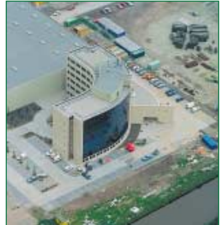
Broad outlook: Econosto's new headquarters in Rotterdam
